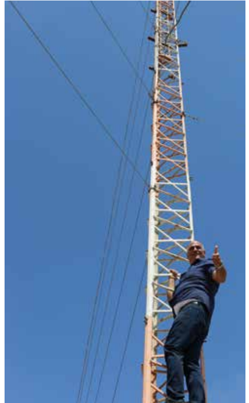
ELIAS CHECKING HIS TOWER OVERLOOKING BETHLEHEM
